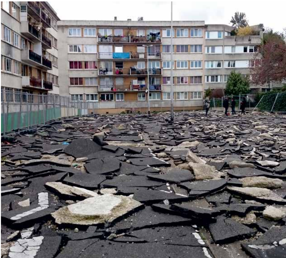
Desealing a car park in Aubervilliers. ©Wagon Landscaping
