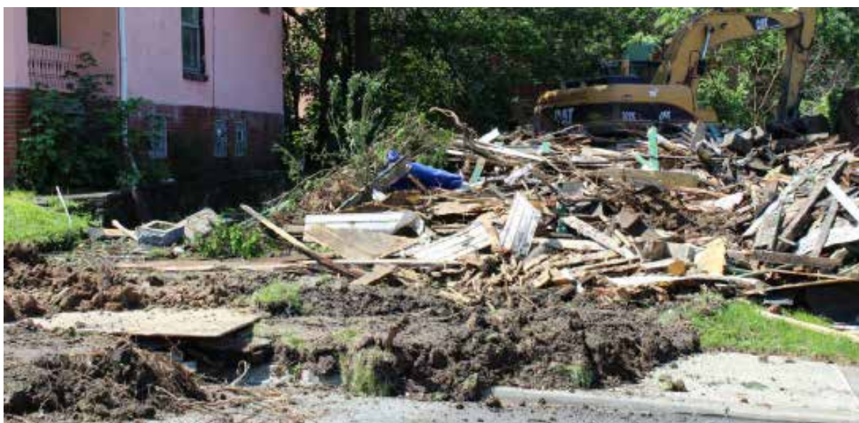
Demolition in Cleveland. ©Turo and Gardiner, 2020 [23]
