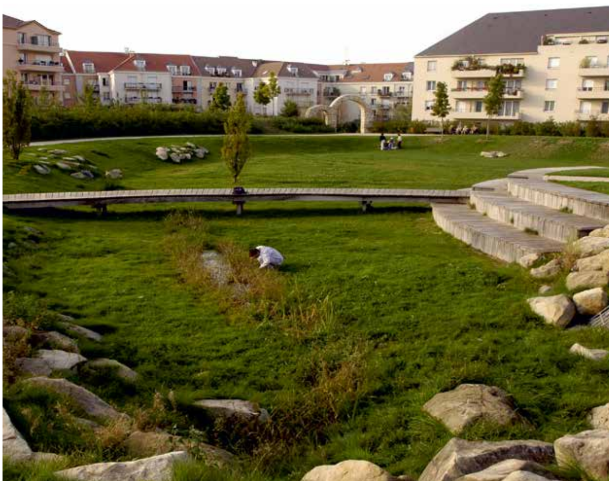
Creation of a floodable parks in the Clos Saint-Vincent district of Noisy-le-Grand ©Département de Seine-Saint-Denis
